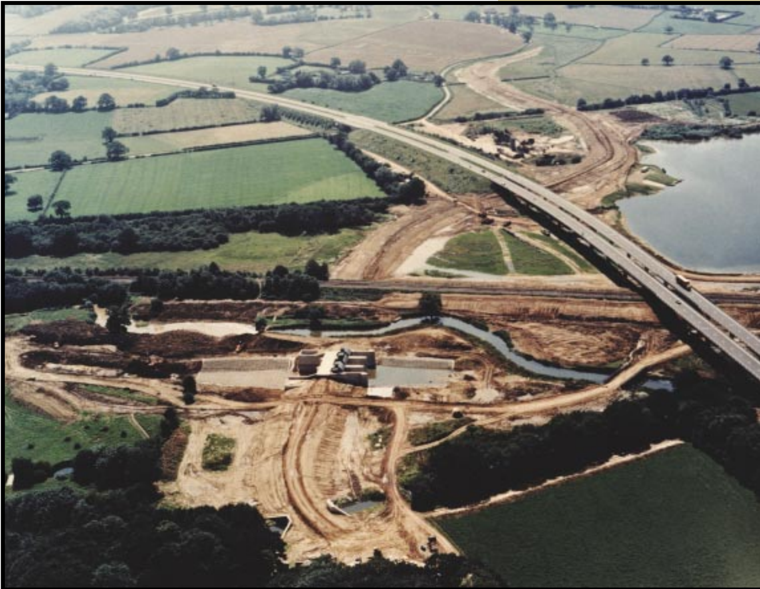
Above: The River Medway was diverted during the summer months while the gates were under construction
